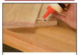
Once all of your holes are drilled apply glue to dowels and you are ready to assemble your joint.
